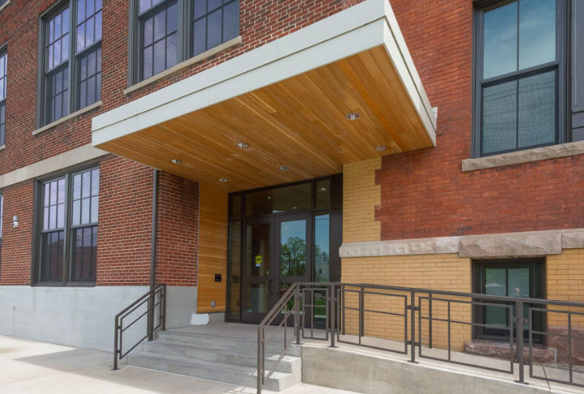
New Front Entrance wood planking provides a warm compliment to existing brick
