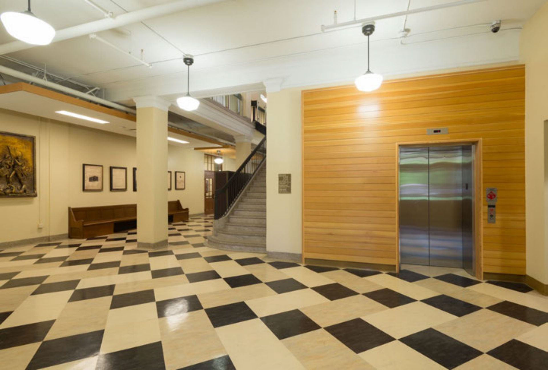
New Elevator constructed in existing light well, elevator avoids taking up valuable floor area
