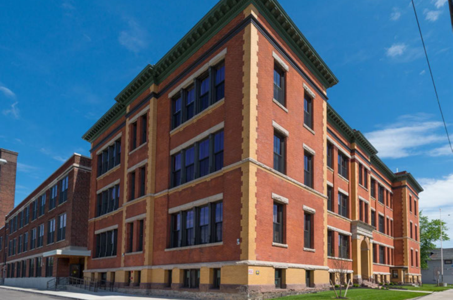
Case Study: DePaul Riverside Apartments
